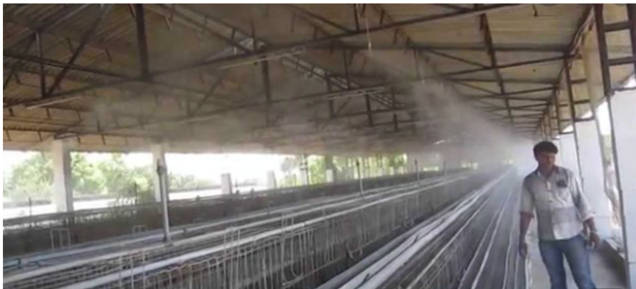
Foggers should mist, not irrigate, and not operate if the humidity exceeds 60%.
